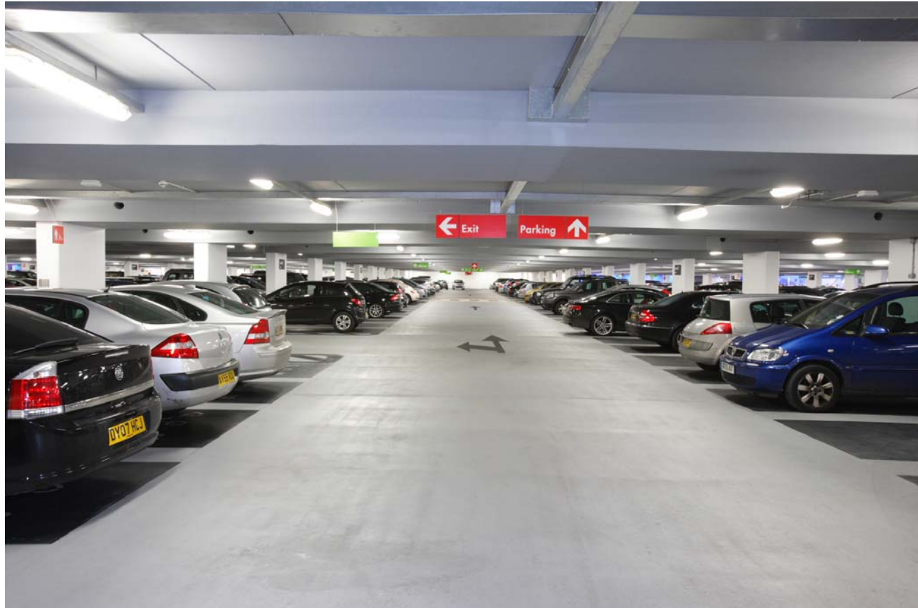
Q-Park Liverpool ONE, Liverpool, UK - New Project
