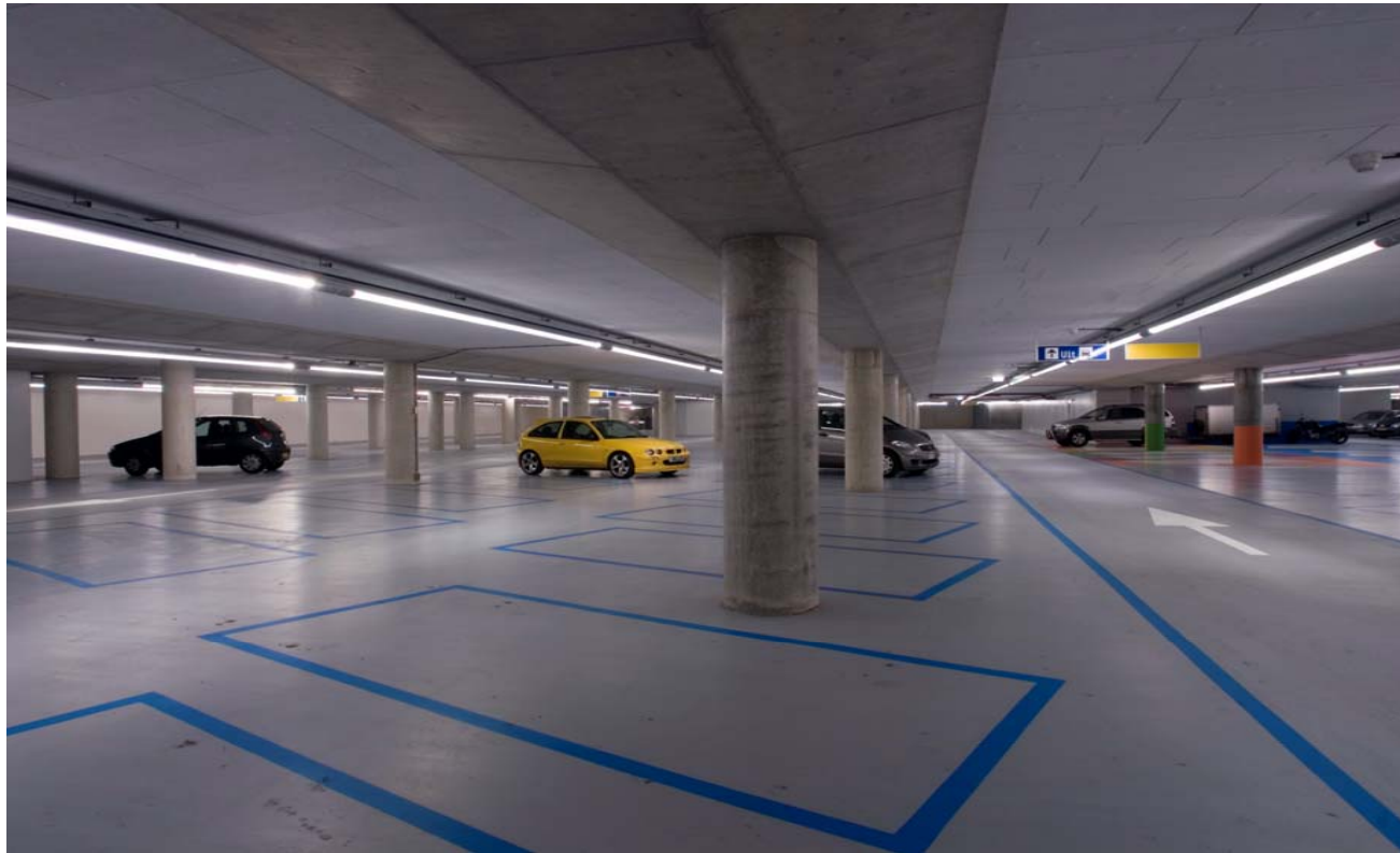
Project; Oosterdokeiland in Amsterdam
